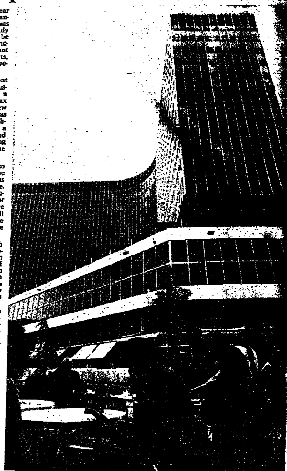
The World Trade Centre, in the Rue l'Évêque, Brussels, a duct of the property boom which has almost come to a halt
